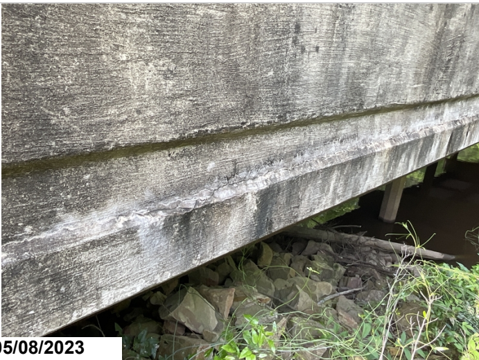
Cracking in parapet wall various locations
