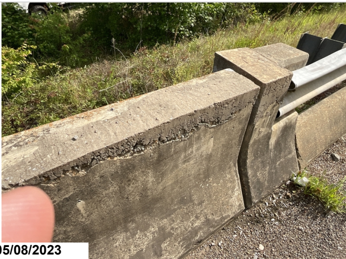
Old patch work on parapet wall various locations
