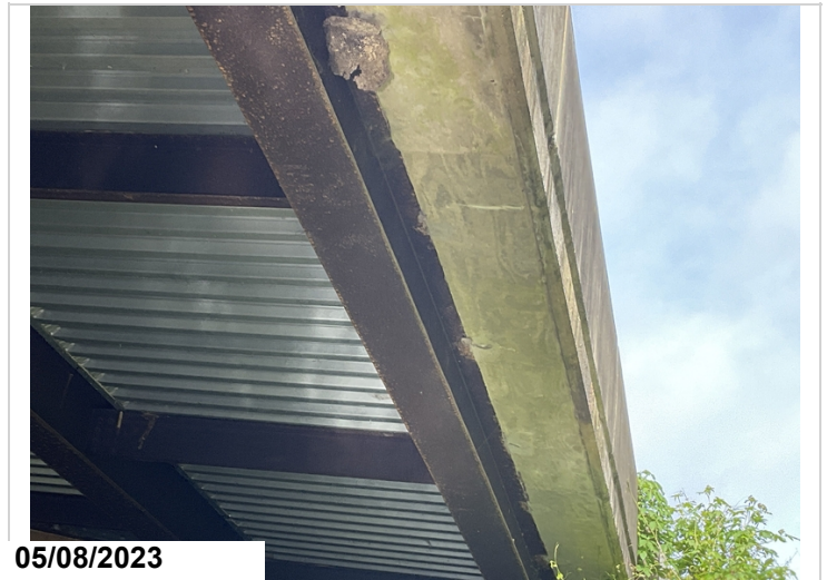
Span 1 efflorescence in overhangs and cracking
