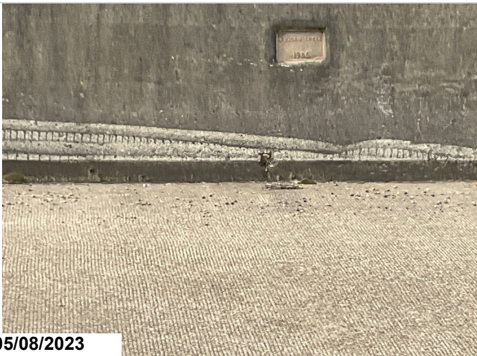
Minor spall in parapet wall various locations
