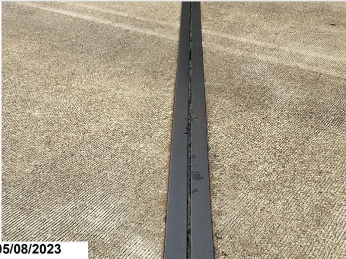
Seal damage bent 6
