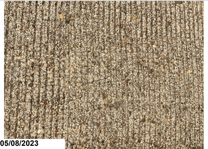
Minor cracking in various locations on deck
