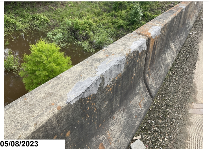
Old patch work on parapet wall various locations
